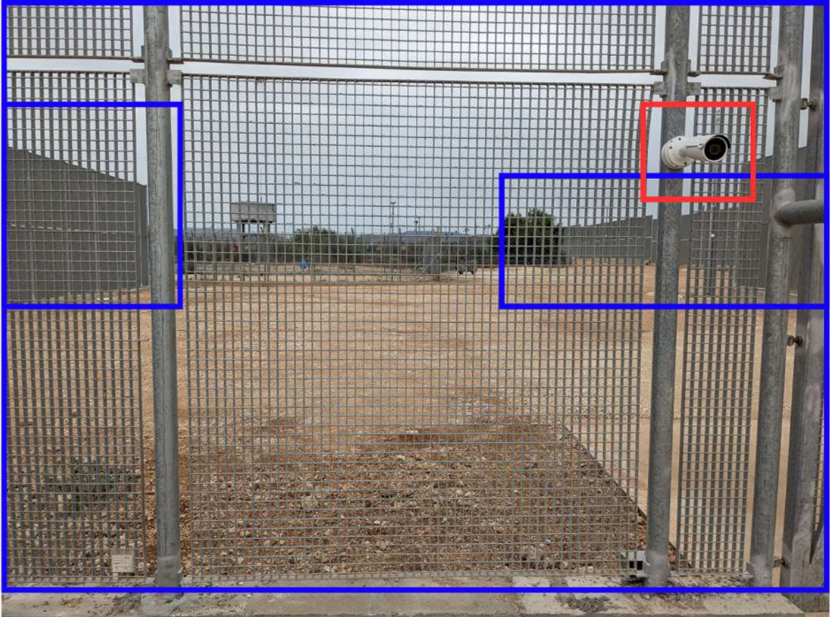
Figure 19: Second perimeter fence and outward facing camera at Pournara (Fencing is marked in blue, cameras in red),12/09/2023, BVMN
