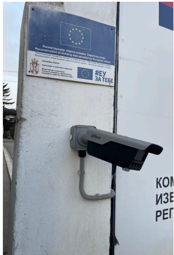
Surveillance Camera in Obrenovac. Source: Collective Aid
