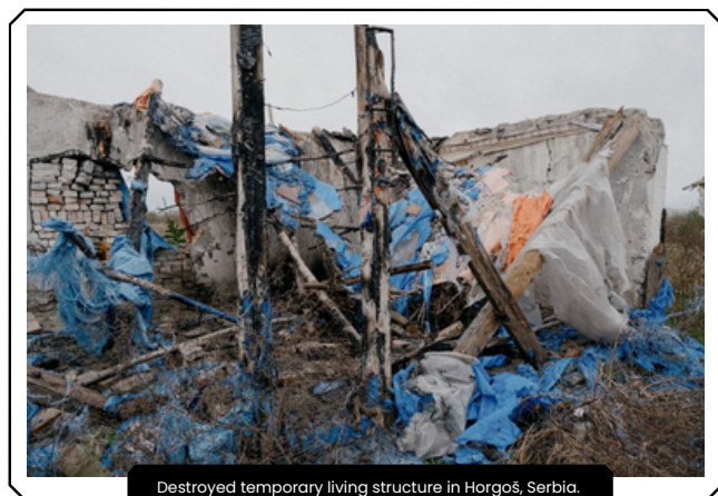
Destroyed temporary living structure in Horgoš, Serbia. ©Collective Aid (Josh Zimmer)
