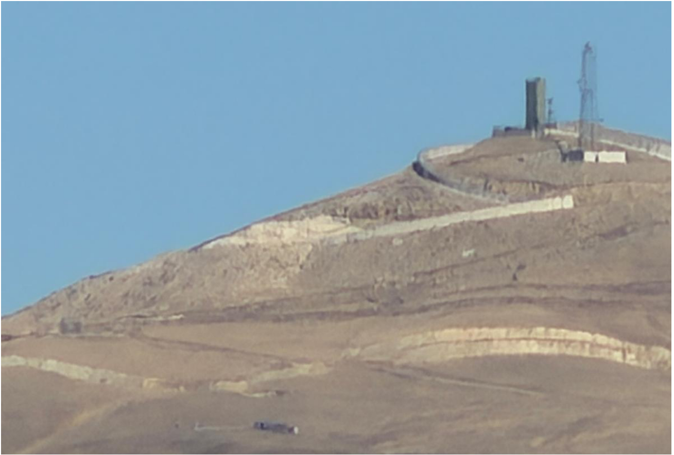
Image 8: An observation tower and electro-optic tower next to each other, Özalp district. Photo taken in November 2025.
