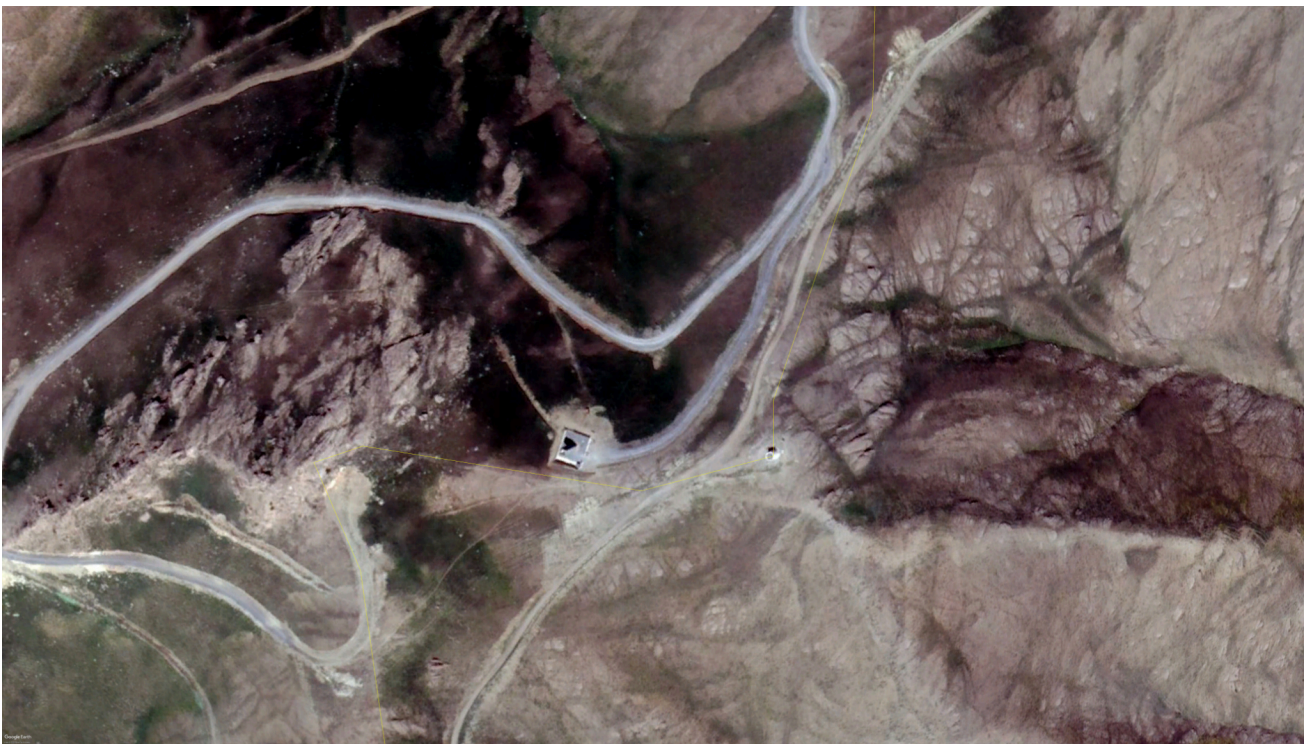
Images 6 and 7: Satellite images showing the construction of an observation tower in 2015 near the village of Mahmutabat, Başkale District. Source: Google Earth Pro. Map data © 2025 MaxarTechnologies.
