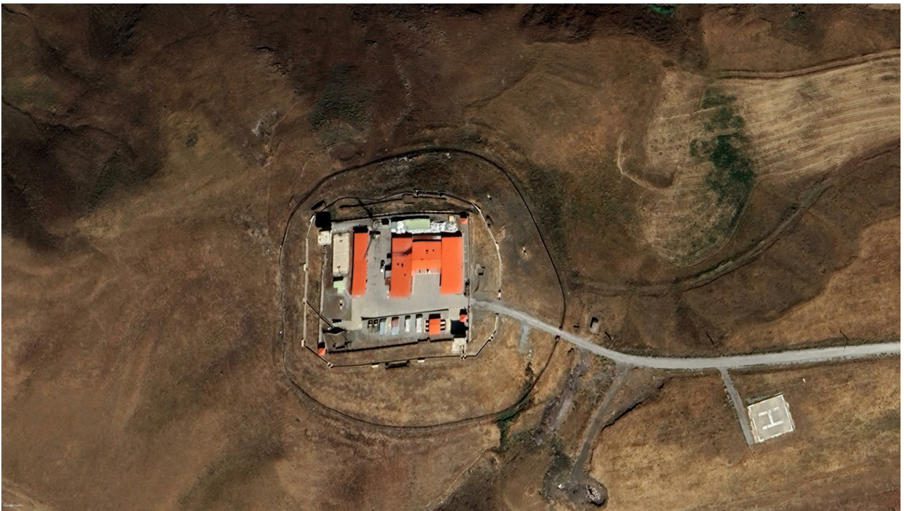
Images 4 and 5: Satellite images showing the construction of a border outpost near the village of Toprakseven in the Çaldıran district between 2010 (top) and 2015 (bottom). Source: Google Earth Pro. Images © 2026 Airbus © 2025 MaxarTechnologies.
