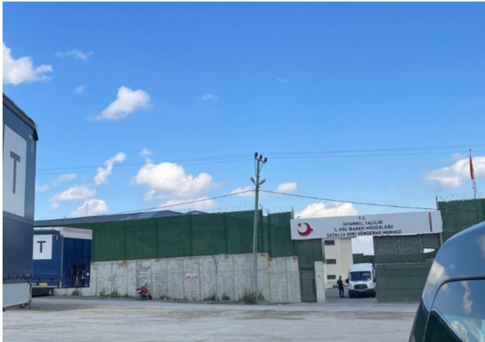
Çatalca İnceğiz Removal Centre. Source: Anonymous
